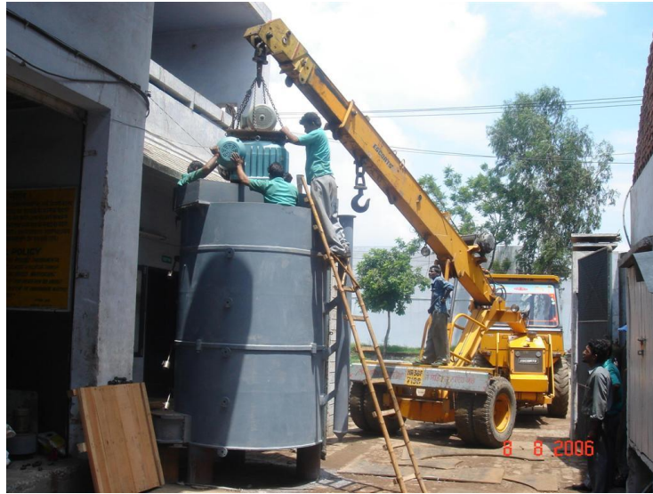
The gear box is being fitted with the help of crane.
